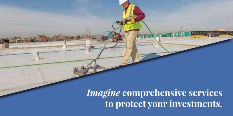
The **RoofTec** High Performance Cleaning System prepares roofs for restoration in record time and is environmentally friendly. By using rotating jets of hot water to carefully and thoroughly scrub the roof surface with a detergent-free cleaning solution that's vacuumed up and removed, rather than run down a storm drain, RoofTec meets both sustainability and labor goals. The result? A superior clean, and roof restoration can often start the same day.
