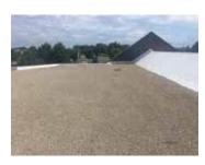
This system has been engineered for great elongation, durability and abrasion resistance. It is waterproof within 30 minutes and can be installed in temperatures as low as minus 20 degrees Fahrenheit. Great in any climate, AlphaGuard PUMA is a perfect choice for installation situations where the air temperature is below 50 degrees.
