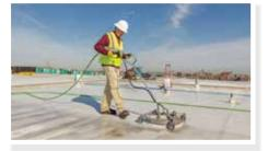
The performance of any restoration coating is compromised when a surface is not properly cleaned and ready for the system application. Not taking care of existing leaks, not replacing wet insulation, using the wrong cleaning system or the wrong cleaning agents, and not allowing time for drying are all contributing factors to a restoration project that will fall short in performance.
