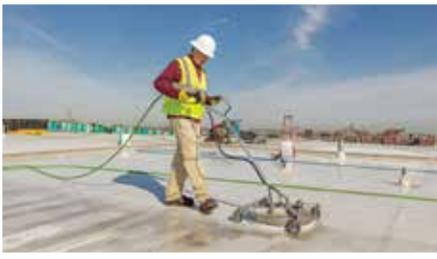
The performance of any restoration coating is compromised when a surface is not properly cleaned and ready for the system application. Not taking care of existing leaks, not replacing wet insulation, using the wrong cleaning system or the wrong cleaning agents, and not allowing time for drying are all contributing factors to a restoration project that will fall short in performance.
